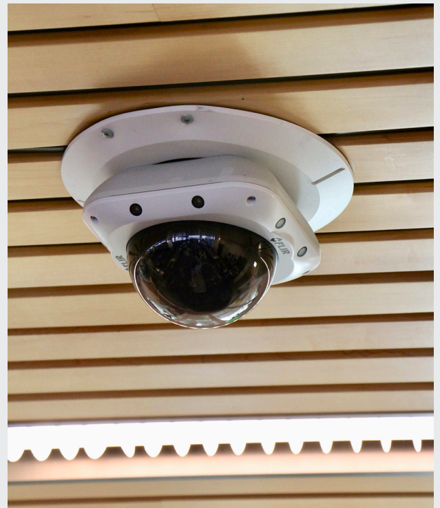
The FLIR Quasar 4 x 2K Panoramic camera is mounted on the ceiling of SJC's TSA checkpoint area to monitor all passenger traffic.
