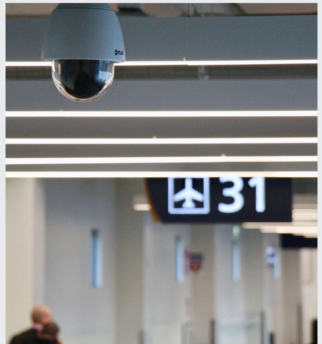
The FLIR Quasar 1080p FHD Dome PTZ camera is mounted within SJC's B Terminal, helping security staff keep passengers and airport personnel safe.
